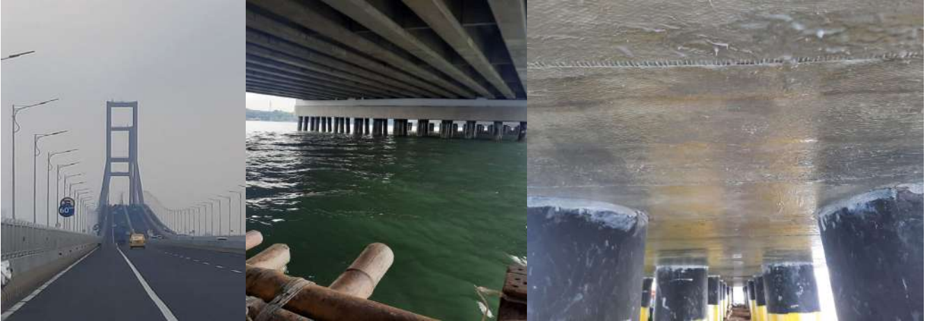
📍 Tol slab repair (Cisumdawu, Lampung-Palembang, Serpong-Cinere)
