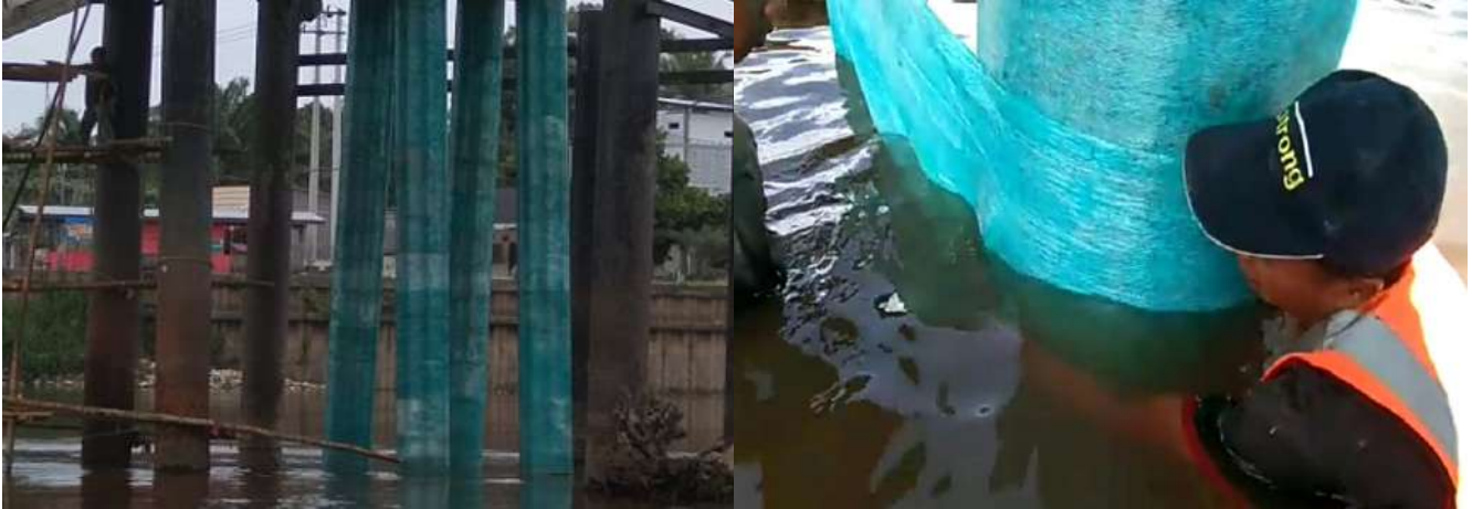
📍 New piles & underwater repair, Coal Jetty, Kintap, Banjarmasin 2019
